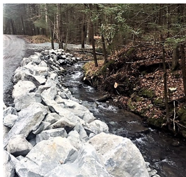
Rip-rap stabilization along a DG project
