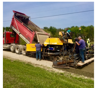
Driving Surface Aggregate (DSA) placement
